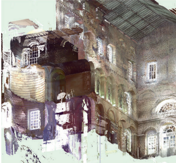
Fig. 14 _ Seaton Delaval Hall | Point cloud capture from three- dimensional site survey scan; detail of main hall and spiral stair.
