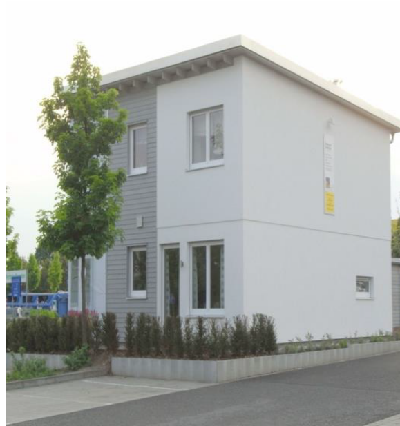
Image.8a (top left and bottom left). The BoKlok standardised elevational panels have been located in external locations that afford ease of removal for access to swap out 'podularisation' or wetrooms and kitchen areas (the areas most likely to require refurbishment)
