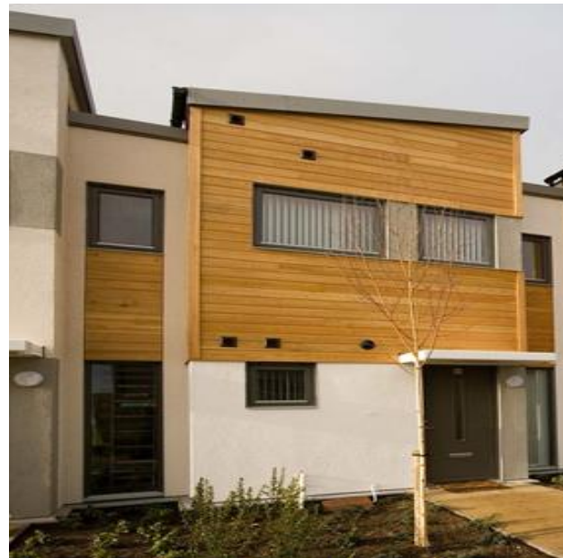
Image.8b. The BoKlok house type shares a standardised format for elevational treatments across all house types. These areas of the façades allow for customized material changes dependent on location of the proposed scheme. The material choice can then be amended to suit local planning requirements, but retain set areas for 'change' that have been detailed to allow for flexibility of fixings for different material choices of rain screen.
