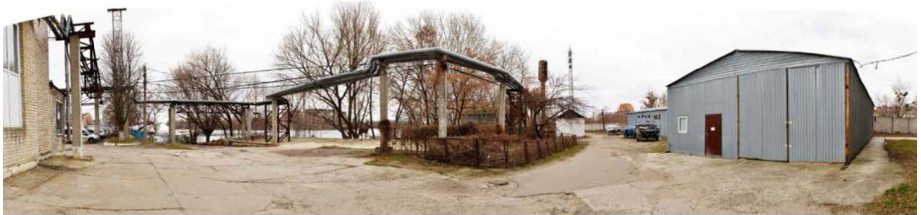
Fig. 01 _ Photos of the site showing the selection of sheds and warehouses from the shipyards
