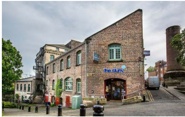
Fig. 26_ Cluny Art Centre within early 19th century warehouse
